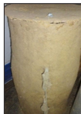
Bamboo storage with mud plaster
